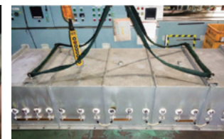
Overhaul according to the maintenance calendar
